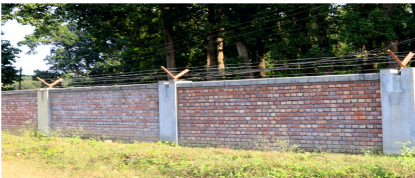
Construction of brick masonry Boundary wall
